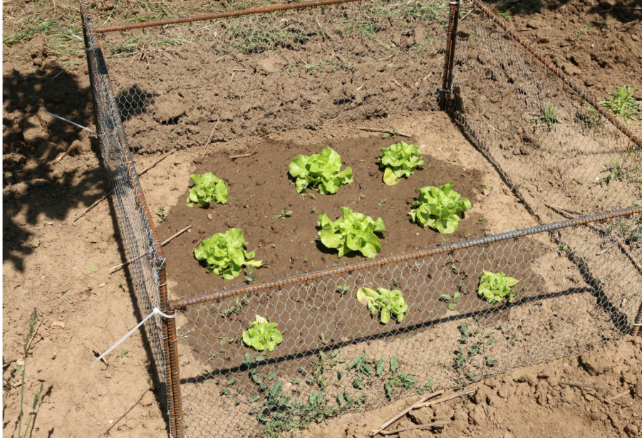
Fig. 1s. Woven-wire, metal-framed fence.
